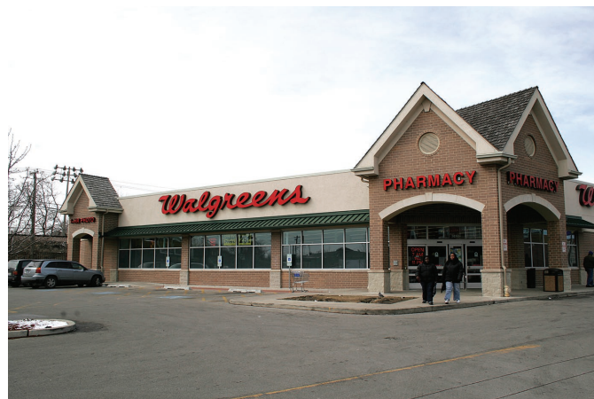
To make their locations more convenient, Walgreens has some freestanding stores not connected to other retailers so the stores can offer a drive-up window for customers to pick up their prescriptions.
